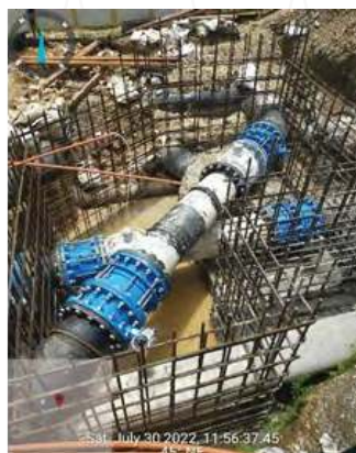
Installation of Flow Meters at Caticlan WTP and Manocmanoc Reservoir
