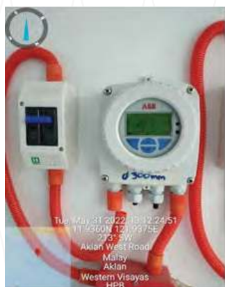
Installation of Flow Meters at Caticlan WTP and Manocmanoc Reservoir
