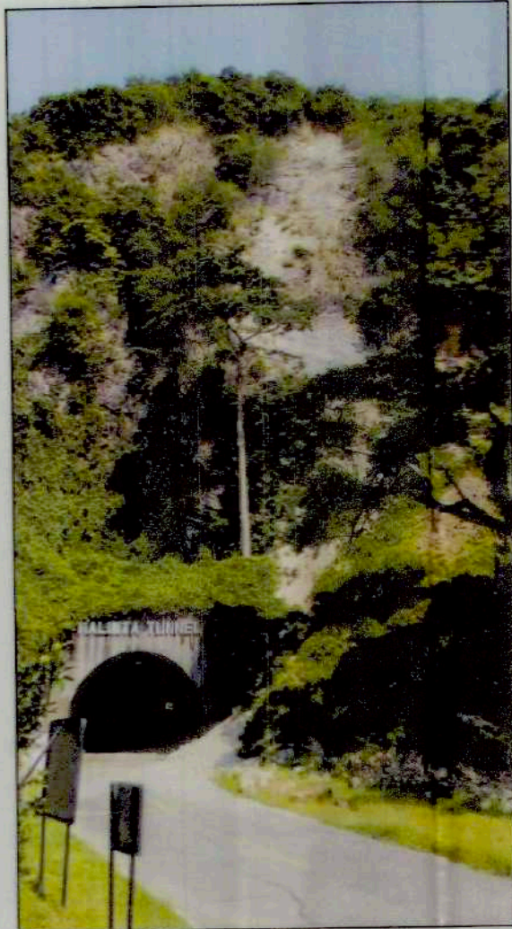
INSTALLATION OF SAFETY MECHANISM / STRUCTURES
